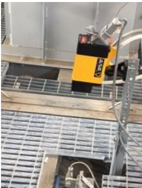
↪ Strip loop control in furnace
